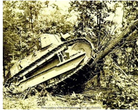
M-1917 modeled on the FT-17, the 6-ton Light Tank was the most numerous tank in the US Army throughout the interwar era, despite its fragility. It could be immobilized by a crowbar.
